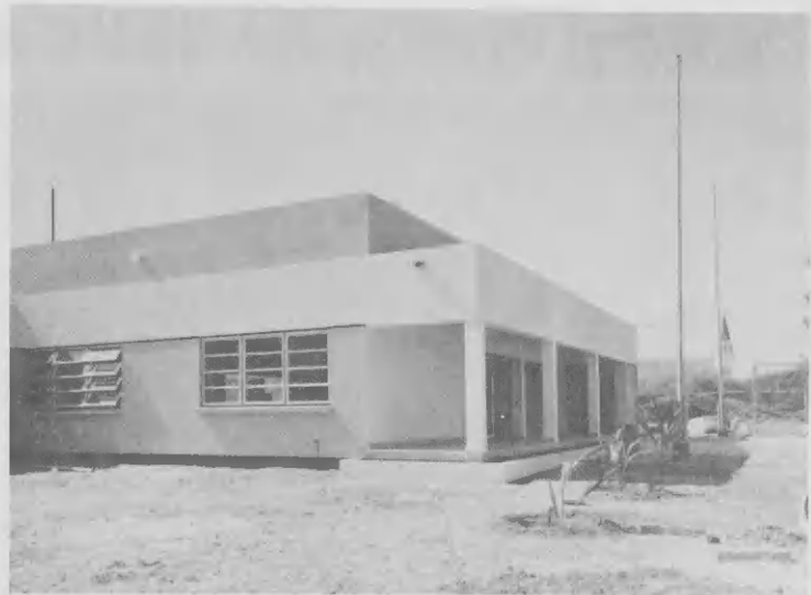
The Noord Community Center is situated on 5000 square meters of land. Notice St. Anne's Church at a distance.
